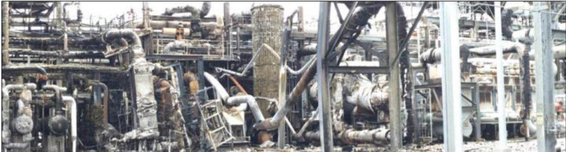
Two separate trains (A & B) after the fire and explosion incident.
